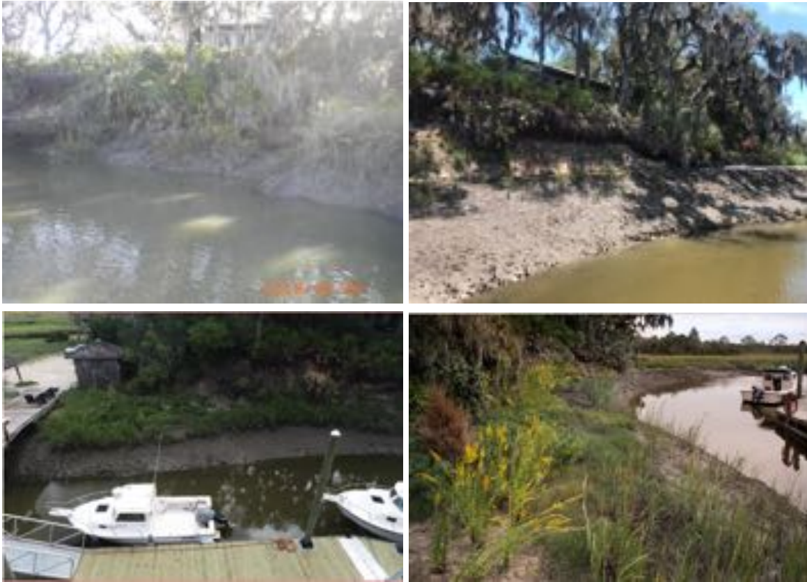
Clockwise, from top left: Pre-construction (February 2018); immediately post-construction (August 2021); post-construction (April 2022); post-construction (August 2022).
