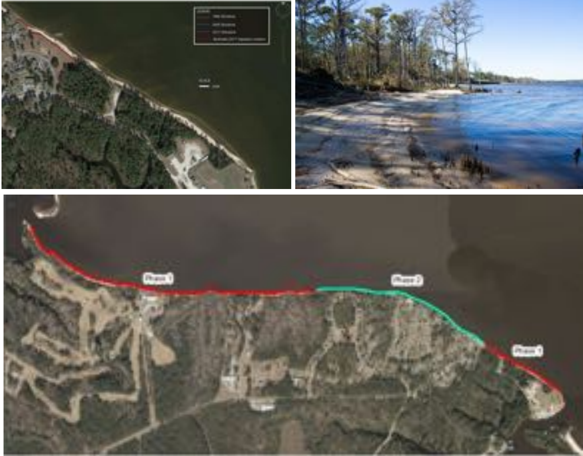
Clockwise, from top left: Aerial view showing shoreline erosion at one stretch of the shoreline; shoreline view showing escarpment and fallen vegetation; initial plans for phased approach, showing overall project footprint. All photos from April 2021 Environmental Assessment and Finding of No Significant Impact.
